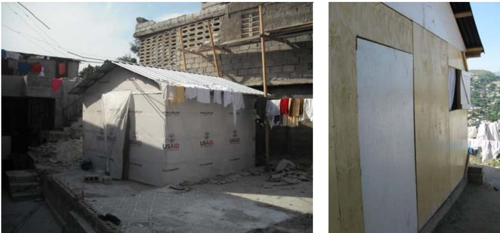
**At left stands a transitional shelter built with plastic sheet walls, no solid doors, no windows, and no foundation. At right, an open window allows air to circulate in a transitional shelter built with plywood walls, doors, windows, and a concrete foundation. (Photos by OIG, November 2010)**
