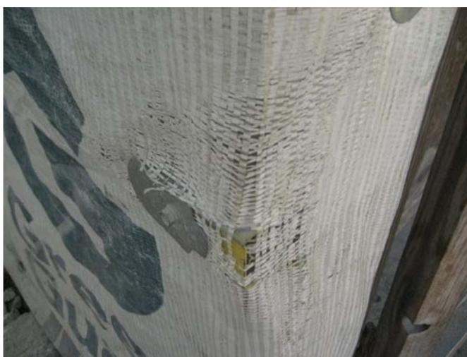
**A transitional shelter constructed with thin plastic sheeting shows wear. (Photo by OIG, November 2010)**
