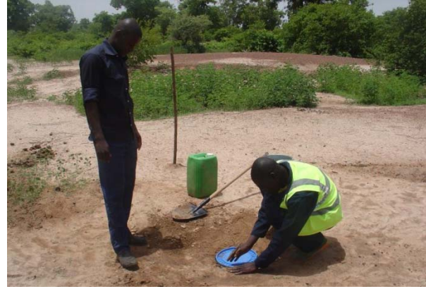
Project staff prepare ground (left) and then install mobile soak pits (right). (Photos by Abt Associates Inc., February 2015)
