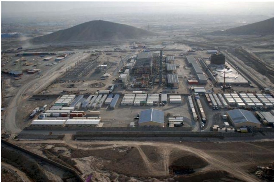
A 105-megawatt power plant in Kabul, built under a USAID/Afghanistan project supported by the Human Resources and Logistical Support Program. The program provides an onsite quality assurance electrical engineer. (Photograph courtesy of Louis Berger Group, Inc./Black and Veatch Joint Venture, October 2009)
