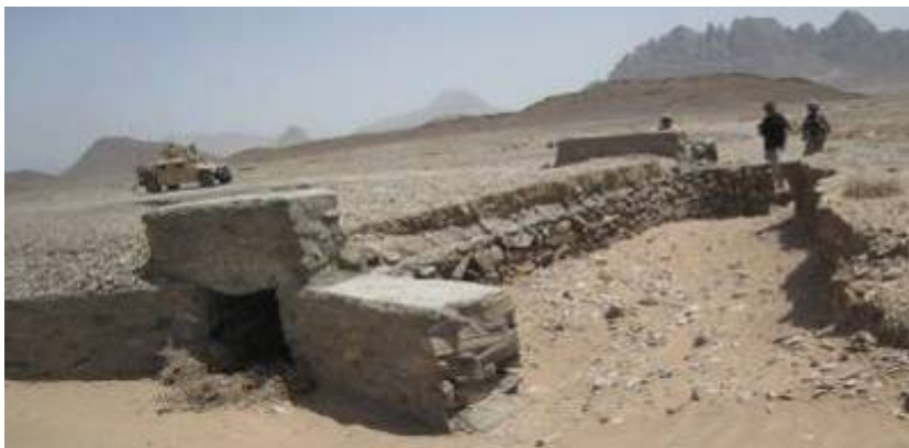
The improper placement of a culvert caused the road to wash out on the USAID-funded Bakwa to Khormaliq road project in Farah Province. (Photograph courtesy of IRD.)
