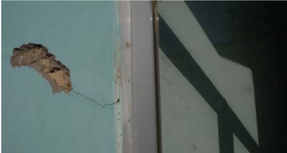
At the agricultural building in Balkh Province, the task force noted major cracks in key locations, indicating that supporting columns are either very weak or nonexistent. (Photograph courtesy of IRD.)
