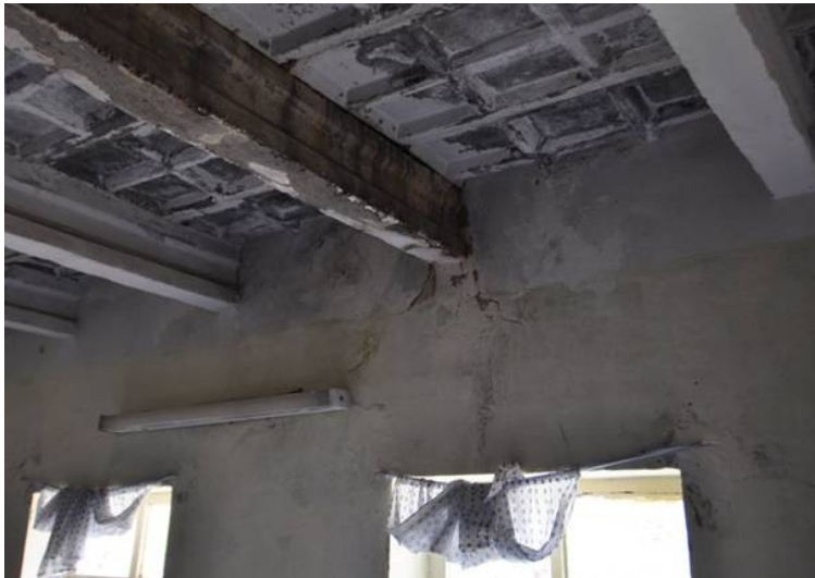
A USAID-built girls' high school in Kabul has unsecured concrete ceiling panels supported by concrete ceiling beams. Signs of stress are evidenced by the cracks in the unreinforced masonry wall. The ceiling panels support several inches of topsoil spread on the roof for insulation. This structural weakness could cause the ceiling to collapse during an earthquake, crushing students under tons of debris. (Photograph courtesy of USAID/Afghanistan.)
