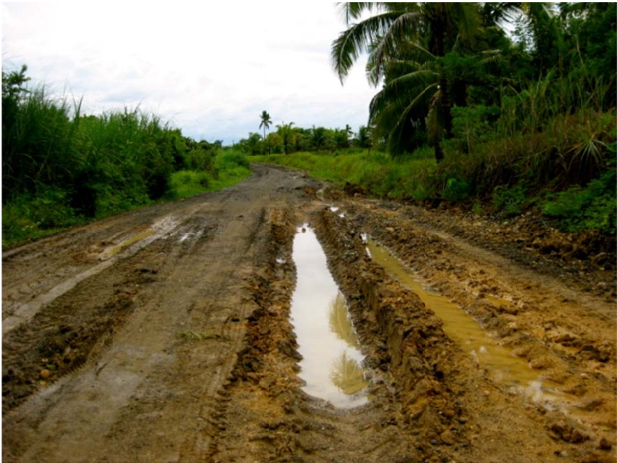
Deep ruts are visible on the newly upgraded Ladia-Raguisi-Pinaring Road only 2 months after its completion in May 2011. (Photo by OIG, July 24, 2011)
