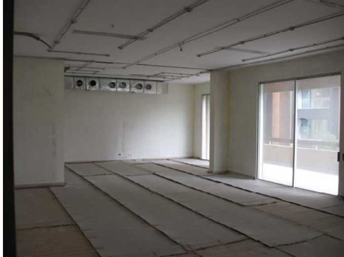
Partial heating and air-conditioning ventilation work begun at the JTI in Beirut, Lebanon. (Photograph taken by RIG/Cairo Auditor, February 2010.)
