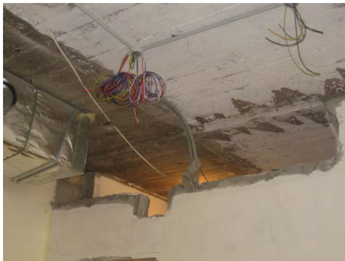
Electrical wiring begun at the JTI in Beirut, Lebanon. (Photograph taken by RIG/Cairo Auditor, February 2010.)
