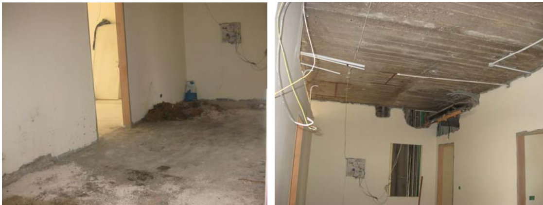
Renovation work begun at the JTI in Beirut, Lebanon. (Photograph taken by RIG/Cairo Auditor, February 2010.)
