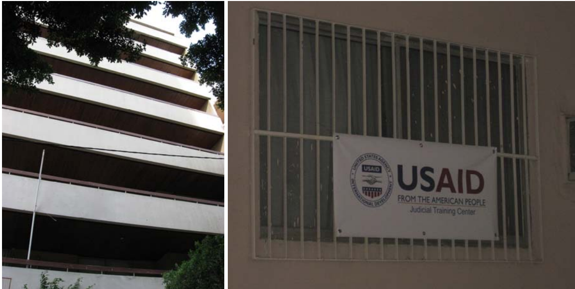
This eight-story building will be used for the Judicial Training Institute in Beirut, Lebanon. (Photograph taken by RIG/Cairo auditor, February 2010.)
