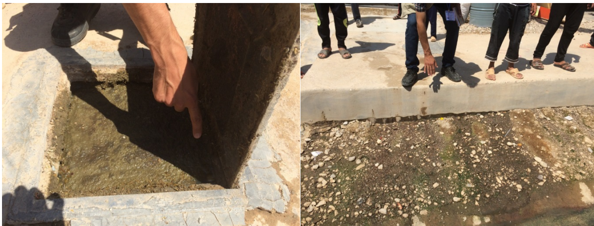
A grant worker points out a full septic tank (left) and sewage seepage (right) at an IDP camp in Ninewa Governorate. (Photos by OIG, July 21, 2015)
