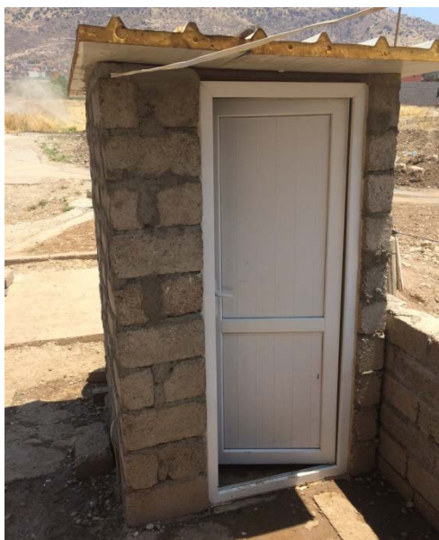
Partners built latrines like this one in Dohuk Governorate. (Photo by OIG, July 21, 2015)
