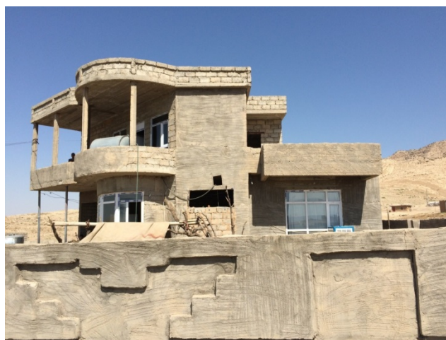
IDPs live in unfinished buildings like this one in Dohuk Governorate. (Photo by OIG, July 21, 2015)
