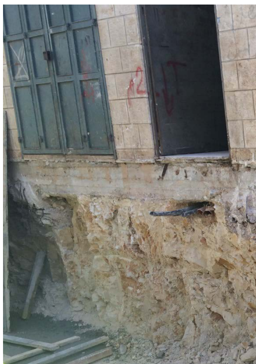
USAID is paying for renovations of the Old Market in Bethlehem. The work includes excavating under an existing building, left, and building foundations (right) for large, metal shade structures. (Photos by RIG/Frankfurt, February 3, 2015)
