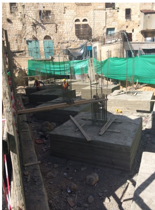
USAID is paying for renovations of the Old Market in Bethlehem. The work includes excavating under an existing building, left, and building foundations (right) for large, metal shade structures. (Photos by RIG/Frankfurt, February 3, 2015)
