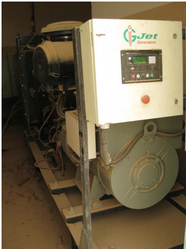
One of two electrical generators, costing $35,500 each, provided under an IRAP grant in connection with an Iraqi rail yard rehabilitation project. Since regional rail service has not yet resumed, operations at the rail yard have been so limited that only one of the two generators was needed; the second one was placed in storage, as shown here. (Photo by OIG.)
