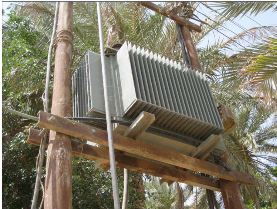
One of the electrical transformers provided under an IRAP grant that has benefited residents in nine villages by increasing their access to electricity. (Photo by OIG.)
