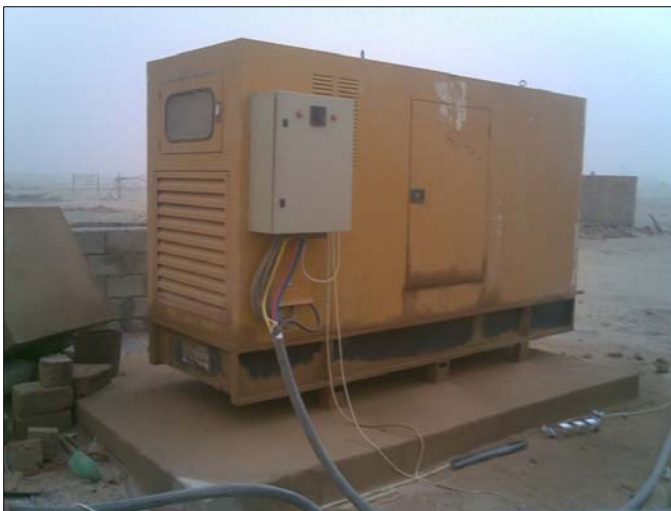
One of two generators installed under an IRAP grant to provide electricity for a university. The grant specifications called for the building of a shelter for each generator to protect them from the elements. However, as this photo reveals, the construction work was not fully carried out, leaving this generator exposed. (Photo by USAID.)
