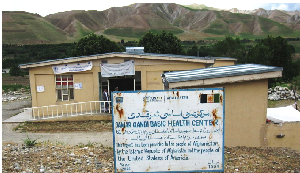
This basic health center in Badakhshan Province serves about 11,700 people. (Photo by OIG, May 9, 2011)
