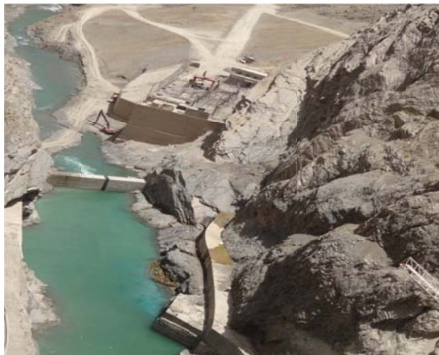
At left is the incomplete switchyard structure. At right uninstalled hydropower components wait inside the structure. (Photos by OIG, June 2012)
