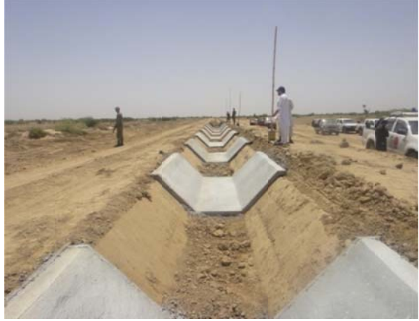
Irrigation work under way includes a barrage for water diversion (left) and canal distributaries like the one above (right). (Photos by OIG, June 2012)
