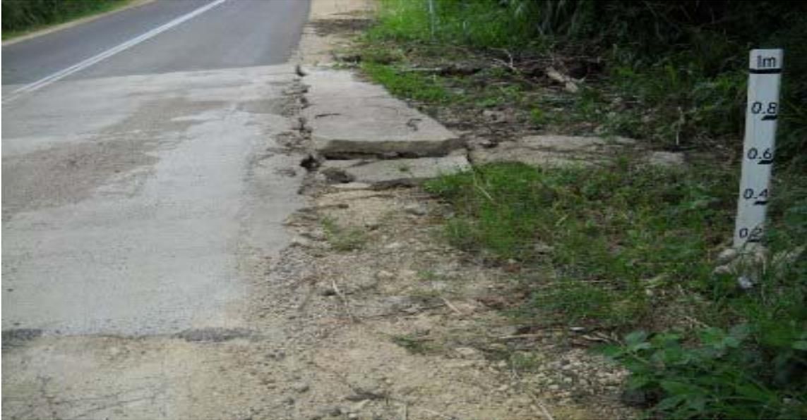
The above photo shows that at the time of the auditors' site visit, a causeway on Efate Ring Road failed after heavy rains. Accumulated rain water found a path under the road. The now unsupported shoulder of the road is breaking up. MCC officials subsequently provided us with a photo showing this causeway has been repaired. See Appendix II. (Photo by OIG, April 20, 2010)
