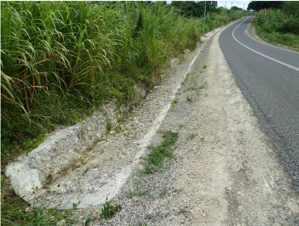
**Figure 2: Photo by Downer 11 September 2010 – Efate Ring Road: Rock Lined Drain (RLD)**
