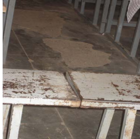
Holes in the floor of a BRIGHT I classroom require maintenance. (Photo by Office of Inspector General, April 2010)
