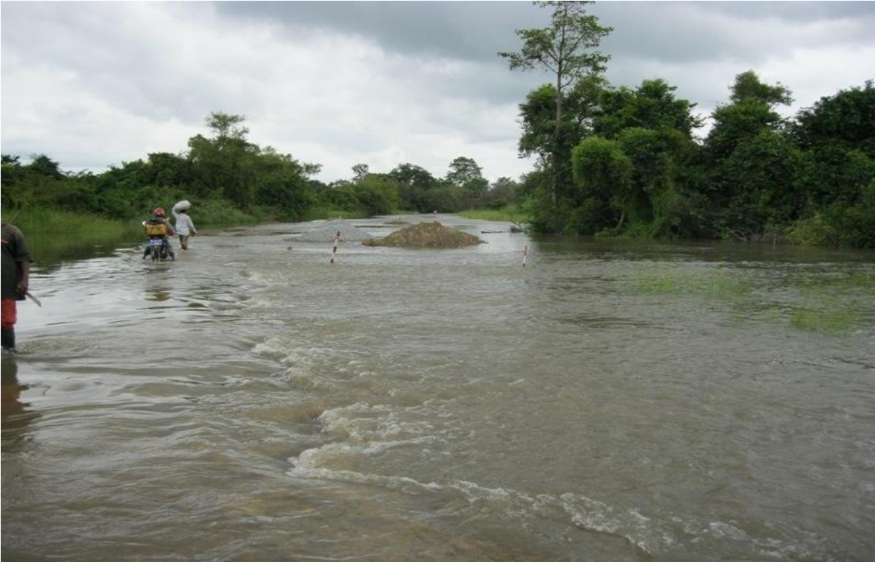
Photo of the AF-2 Trunk Road underwater in Ghana. (Photograph by MiDA's procurement agent.)
