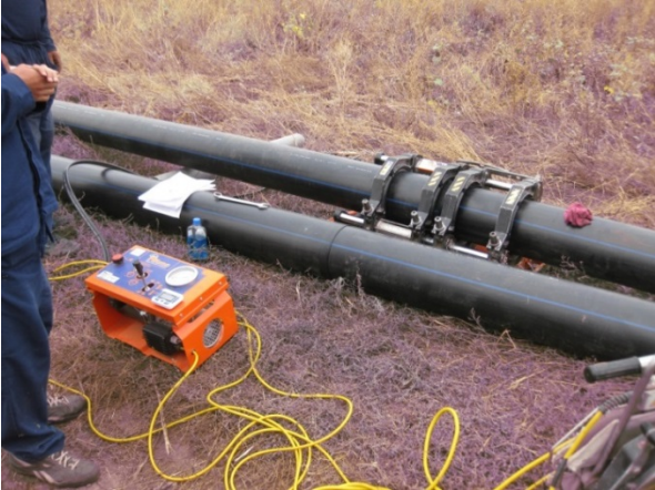
Workers use heat fusion to join replacement pipe sections. (Photo by OIG, September 2013)
