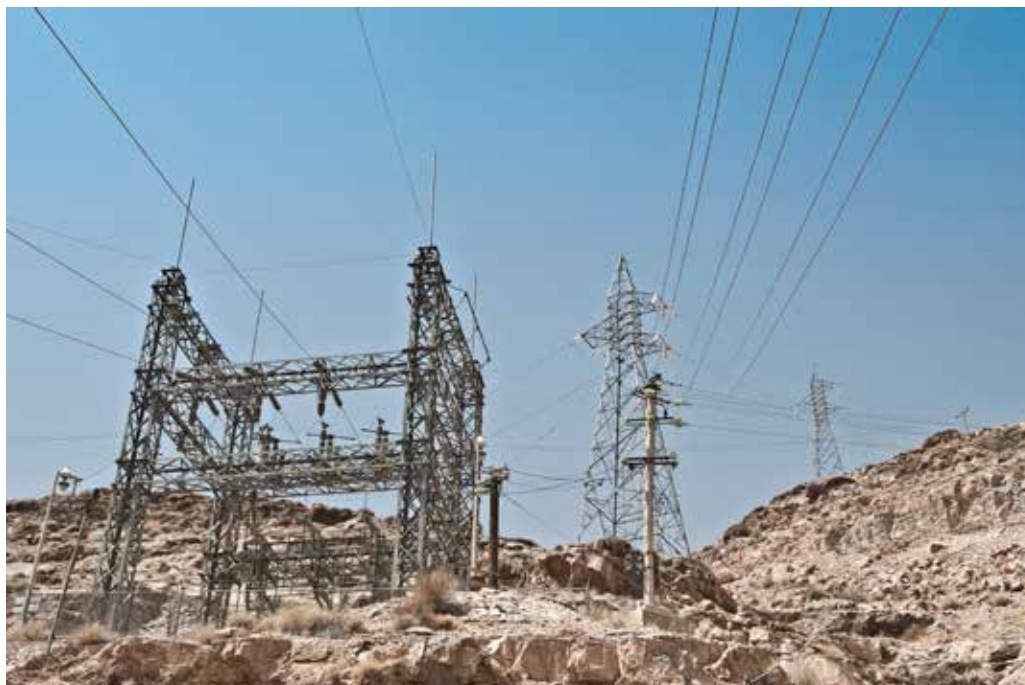
A series of power lines and substation connected to the Kajaki dam's hydroelectric power plant. (U.S. Navy photo)
