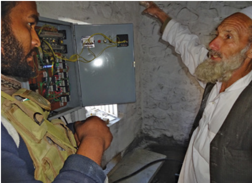
An Afghan local conducts a maintenance assessment validating his understanding of the power plant’s operational and sustainment requirements. (U.S. Army photo)
