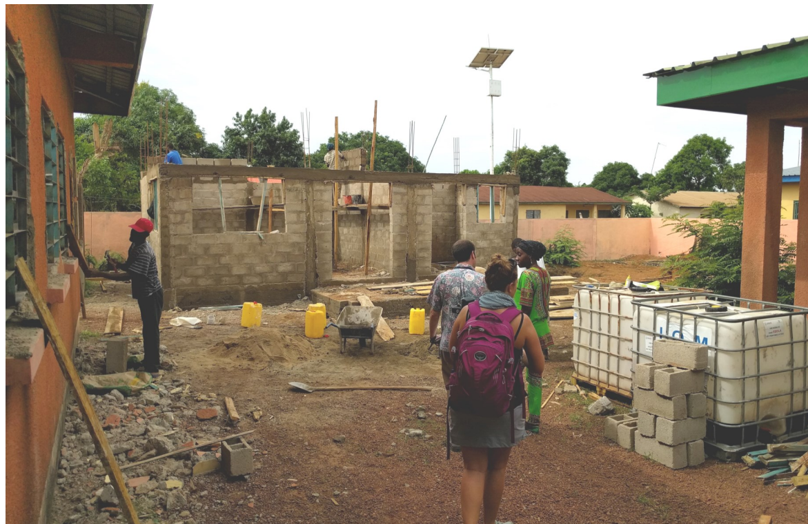
USAID team inspecting a health center under renovation in Forecariah, Guinea. (Source: USAID OIG, June 13, 2016)
