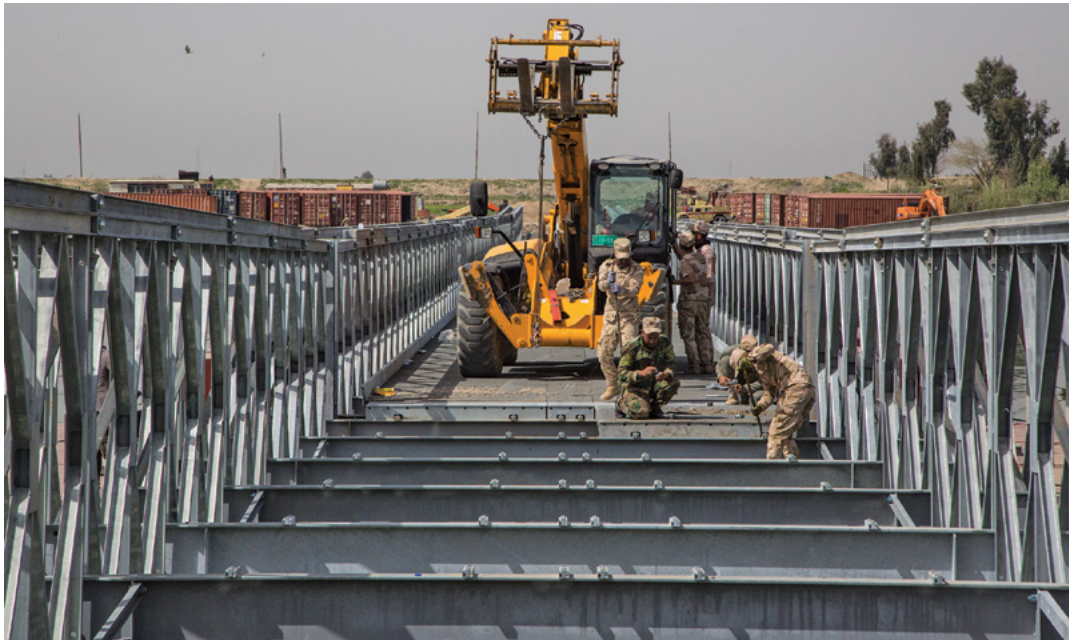
The United Kingdom Bridge Training Team advises and assists Iraqi security forces in construction of an Acrow Poseidon bridge over the Tigris River in Mosul, Iraq. (U.S. Army photo)
