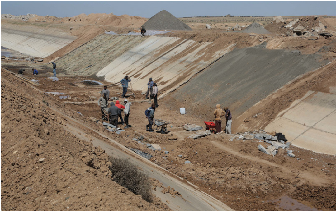
Workers shovel dirt and lay rebar to restore part of the canal in Shanena, Syria. (U.S. Army photo)
