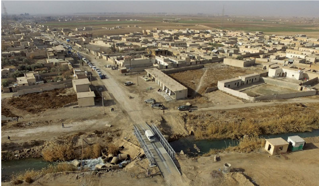
Engineers attached to the Special Operations Joint Task Force-OIR erected a bridge over the Euphrates River in the Raqqah district, Syria. (Special Operations Joint Task Force-OIR photo)
