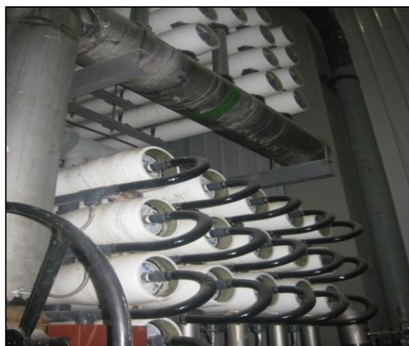
Water passes through reverse osmosis membranes that are used to remove dissolved impurities from water at the Zara Ma'in Desalination Plant (photo by OIG).
