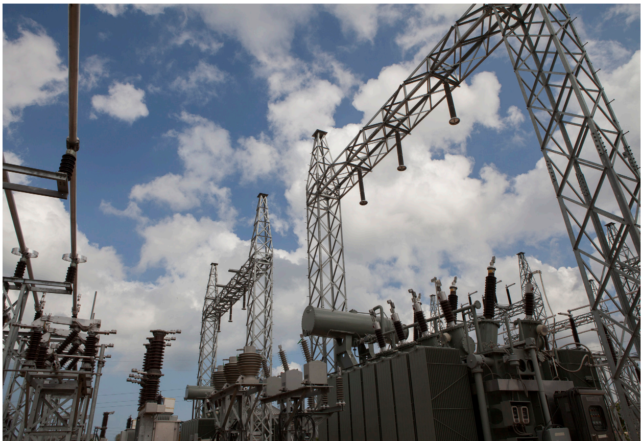
Pictured above is the MCC-funded Mtoni Service Station on the Zanzibar Archipelago. (Photo by Jake Lyell for MCC.)
