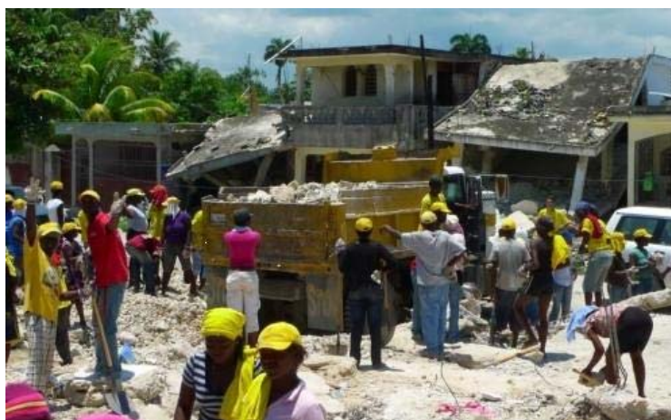
To remove rubble, the implementing partner used small labor teams to supplement heavy equipment. (Photo by implementing partner.)
