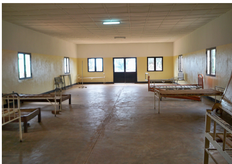
This ward in Muyinga Hospital was not being used because a USAID funded program did not deliver beds and mattresses on time (photo by RIG/Pretoria).
