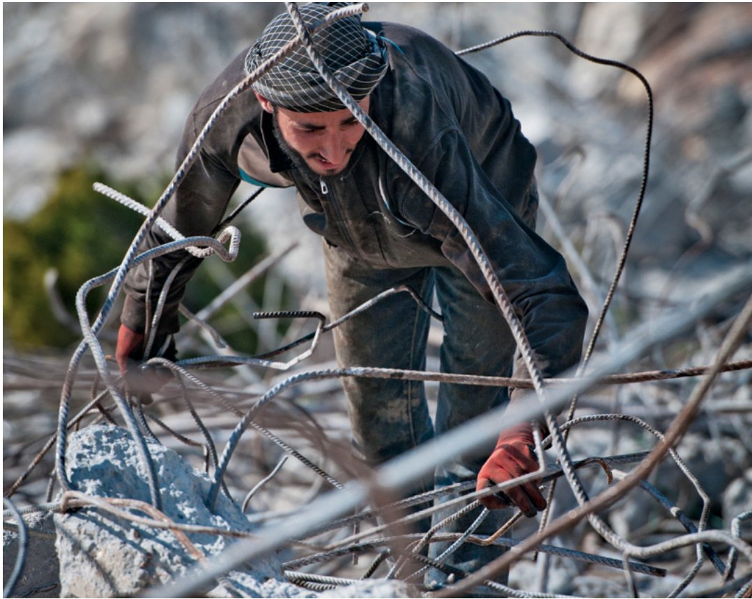
A man scavenges rebar from a destroyed building in Raqqah, Syria. (U.S. Army photo)
