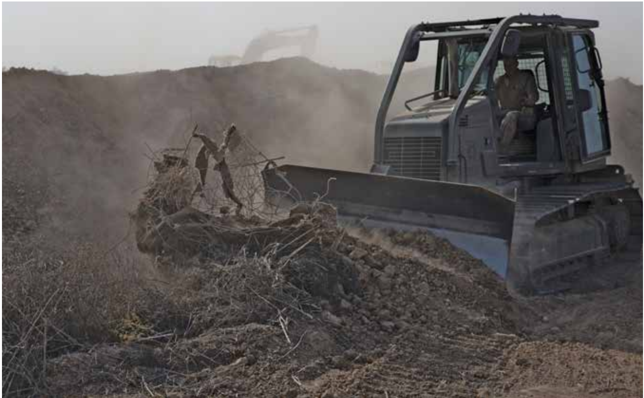
Spanish and Iraqi soldiers build improvements on a bomb disposal school at the Besmaya Range Complex, Iraq. (U.S. Army photo)
