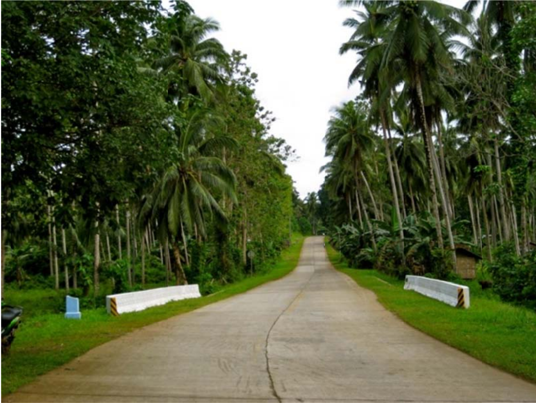
The Bañas Bridge, a box culvert bridge, is situated along a remote section of a rural highway on the island of Basilan. (Photo by OIG, July 16, 2011)
