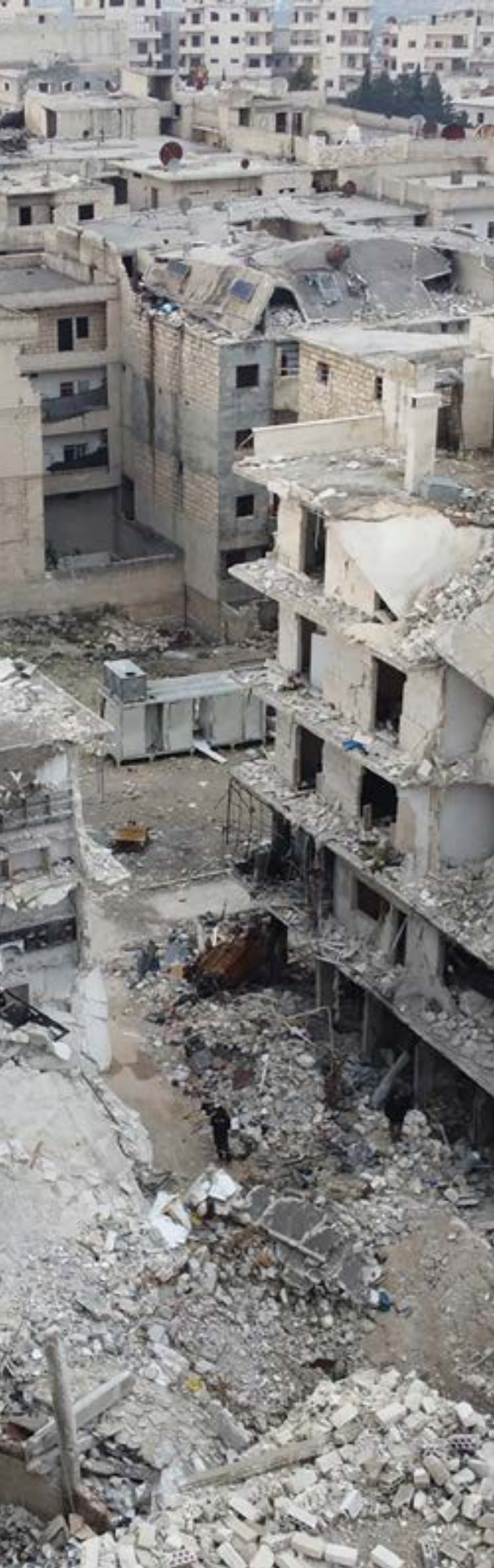
Escalating levels of conflict destroyed buildings in Idlib Governorate, Syria. (WFP photo)
