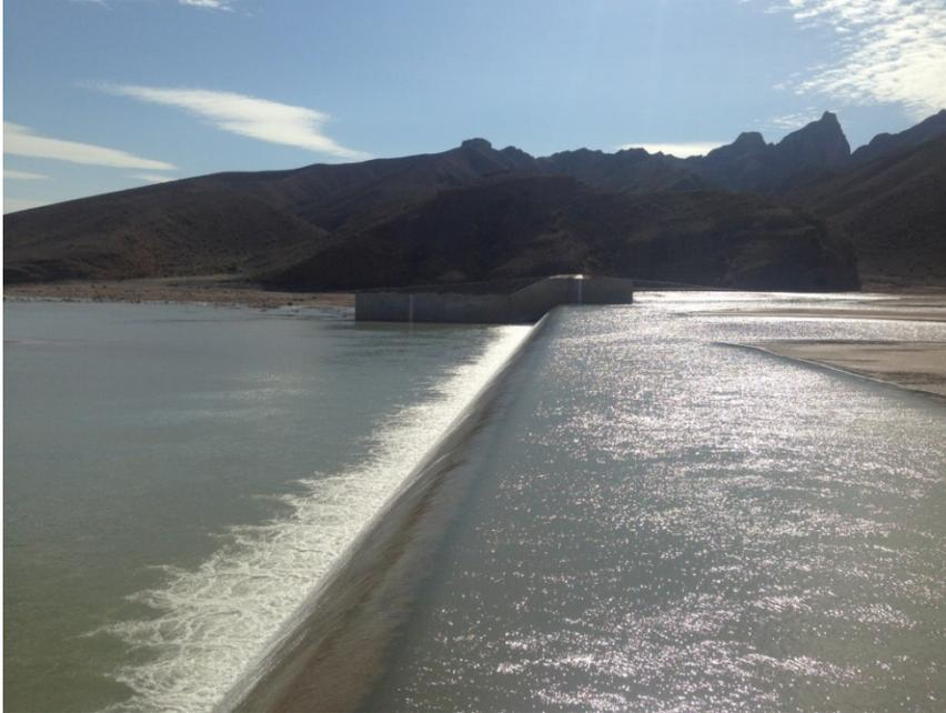
*The barrage at the mouth of the dam diverts water to the main canal.*
