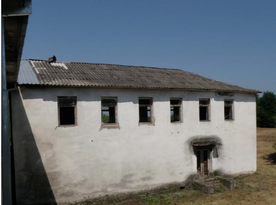
The roof of the Kuchatani school's attached gymnasium is made of asbestos-containing materials. Renovations were made to the connecting segment (shown at left), but not to the gym's roof. (Photo by OIG, July 27, 2011)
