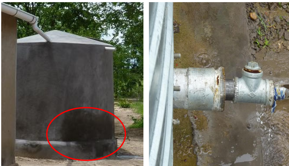
The rainwater harvesting tank at left, built by Adventist Development and Relief Agency International, did not cure properly and shows water seeping through the side. The school rainwater harvesting tank at right, built by Medair International, has a broken tap. (Photos by RIG/Pretoria, Gokwe North District, January 26-27, 2012)
