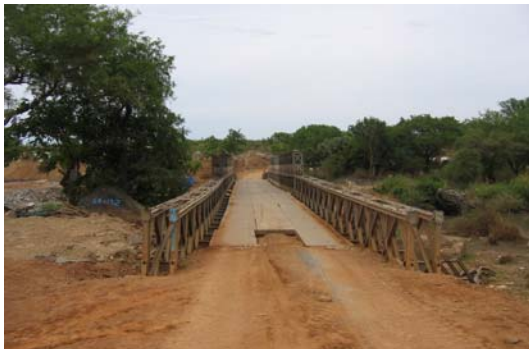
The photograph on the left is of an existing, repaired Bailey bridge; the photograph on the right shows one of the new bridges. Both photographs taken on the Juba-Nimule road. (Regional Inspector General/Pretoria, April 28, 2009.)
