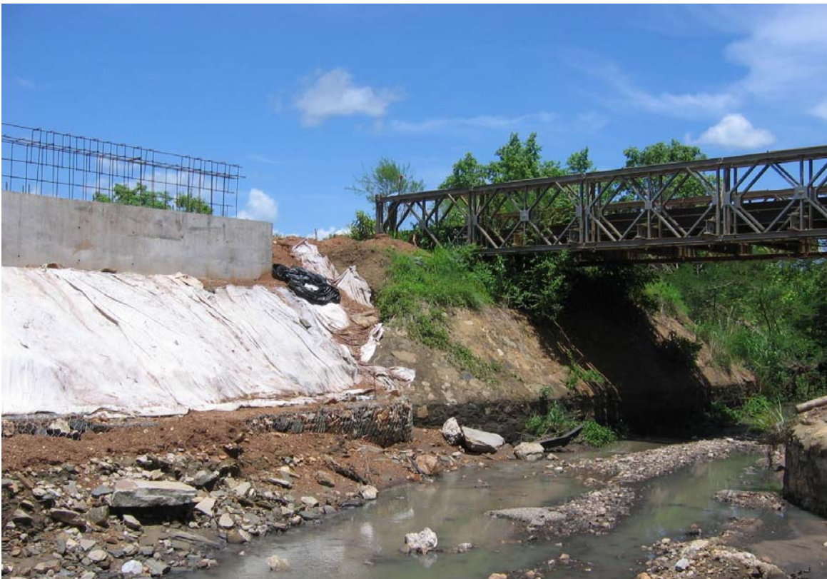
Photograph of a Bailey bridge on the right with abutment for the replacement bridge being constructed on the left. Photograph taken on the Juba-Nimule road. (Regional Inspector General/Pretoria, April 28, 2009.)
