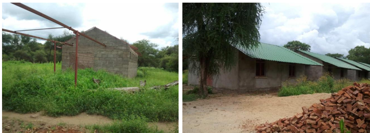
The Mabaan County vocational training center, constructed under MC-BRIDGE, is incomplete. The structure on the left is an unfinished dormitory. On the right, a dormitory does not have windows or flooring yet. (Photos by Mercy Corps, September 2011)
