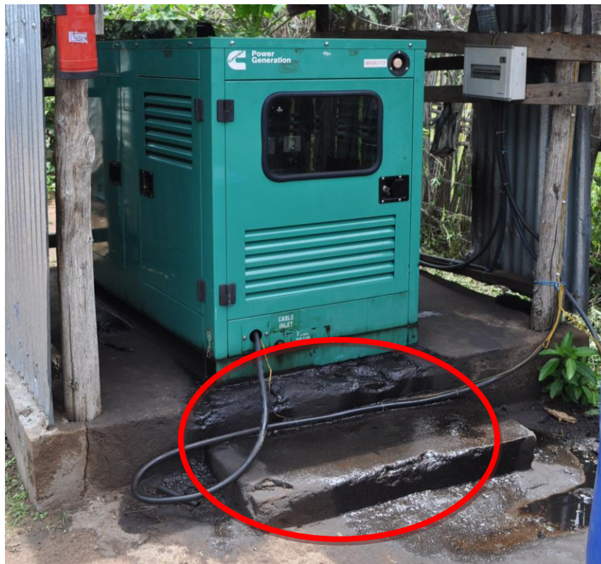
The generator at the Lainya resource center has an oil leak (circled) and works sporadically. (Photo by RIG/Pretoria, August 2011)
