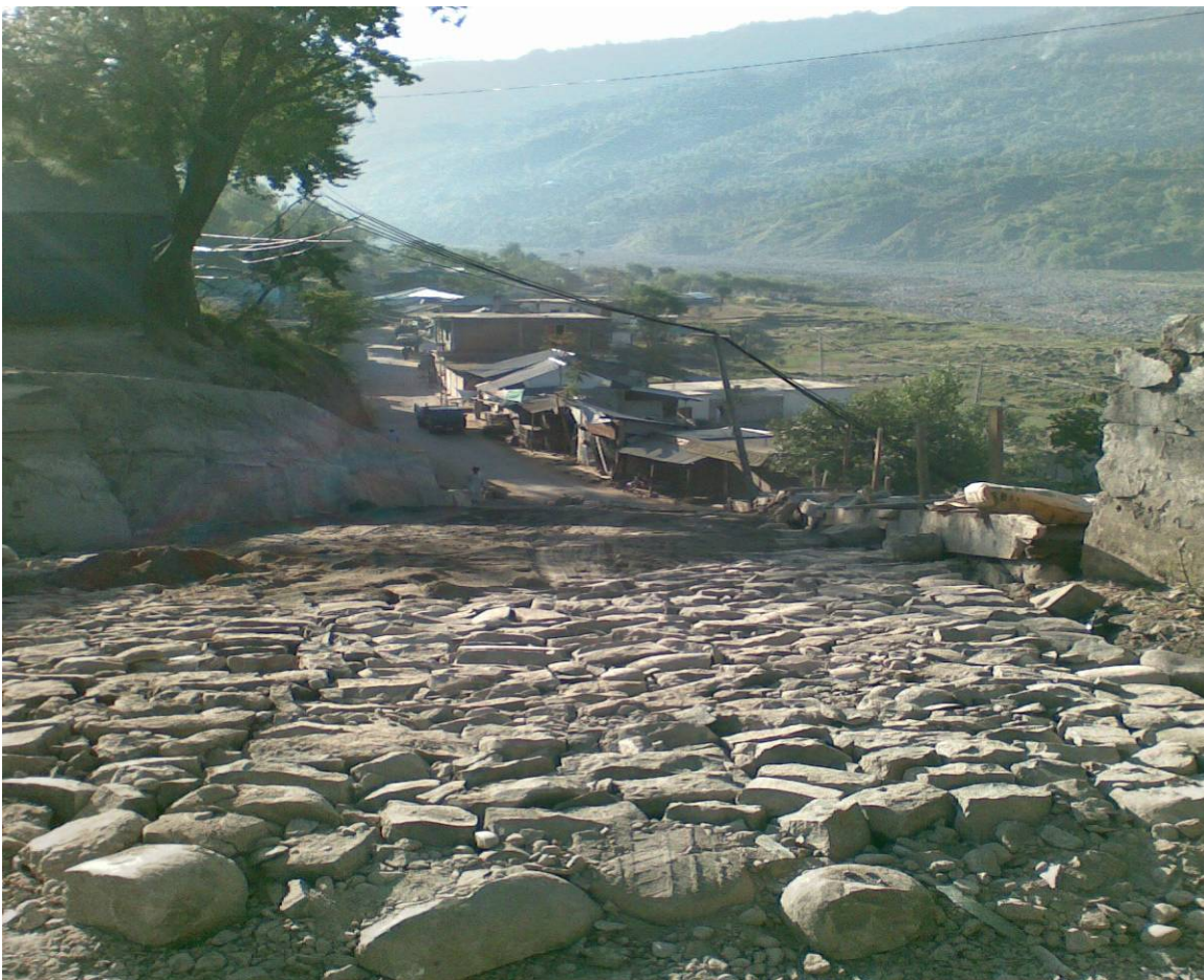
To provide better access to the Chatter Health Care Facility in the Bagh District, a small grant was approved by the health management committee for this new road, shown here under construction. (Photo by Office of Inspector General, November 2009.)
