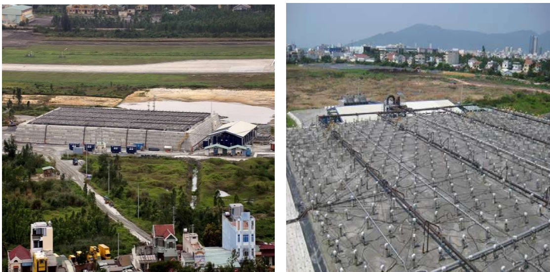
USAID funded an IPTD treatment facility (left) that uses heating wells (right) to remove dioxin from soil and sediment. (Photos by Tetra Tech Inc., February 12, 2014, and Terra Therm Inc., April 23, 2014)
