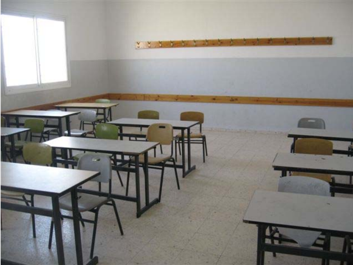
Classroom constructed at Wadi Fukin school in the Bethlehem Governorate under the Emergency Jobs Program. (Photo by Office of Inspector General, June 2010)
