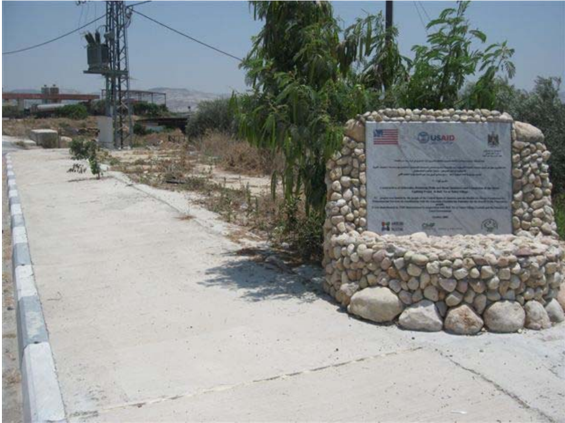
Emergency Jobs Program plaque stands alongside the Beit Ur Al Tahta sidewalk project in the Ramallah Governorate. (Photo by the Office of Inspector General, June 2010)
