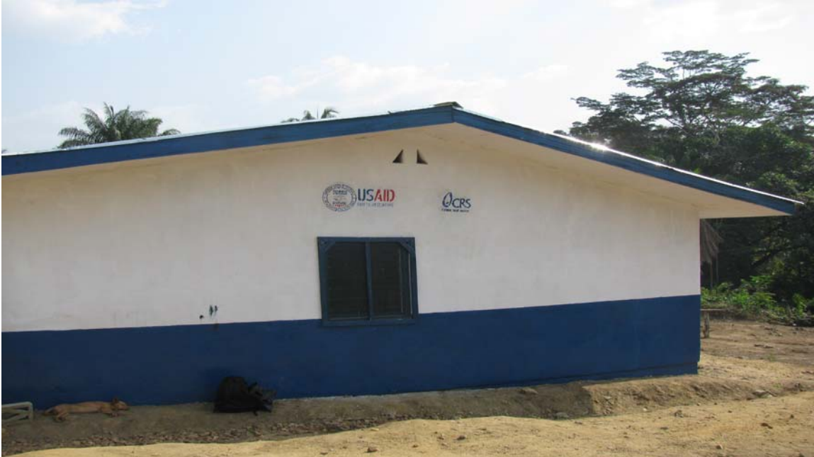
A rehabilitated clinic stands in Gbanla Town, Bong County. (Photo by an Office of Inspector General auditor, January 2010)
