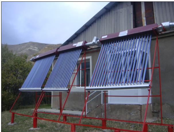
Some of the projects USAID funded under Task 2 included equipping a medical clinic with a solar air heating system (left) and replacing a village's corroded steel and cast-iron water pipes (right) with ones made of polyethylene. (Photos by OIG, October 2013)
