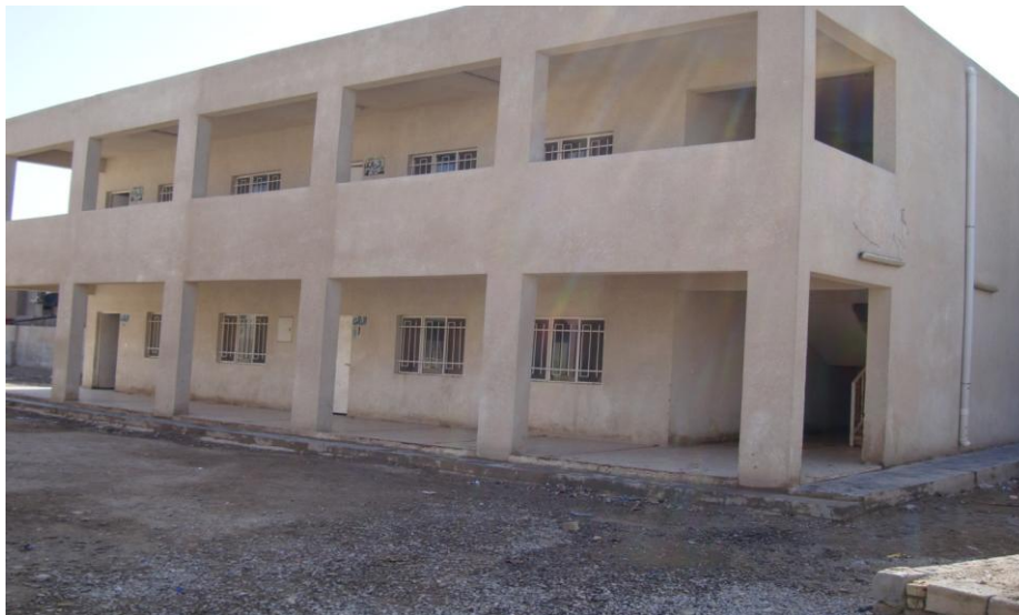
IRD's subcontractors built these classrooms at a primary school in Baghdad. (Photo by Combined Consultancy Company for Legal and Economic Investment Consultation, LLC, of Karradah, Baghdad, under contract with OIG, April 2011)
