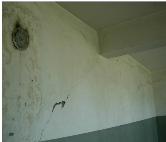
This wall in the Sherzad Girl's School shows vertical cracks caused by the earthquake. (Photo courtesy of USAID/Afghanistan)
