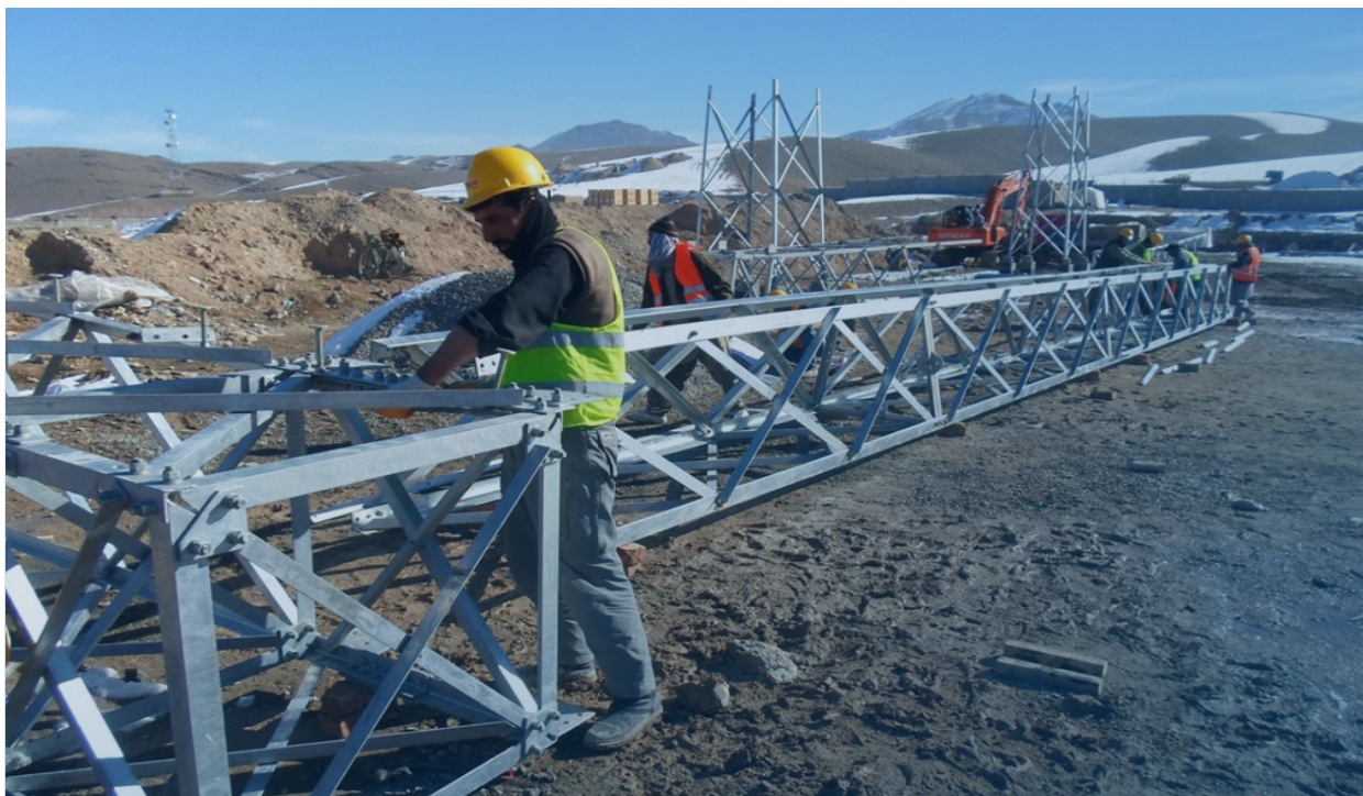
Workers install the equipment to erect an electricity tower linking Kabul to Kandahar and Helmand, Afghanistan. Photo: USAID/Afghanistan (Jan. 17, 2016)
