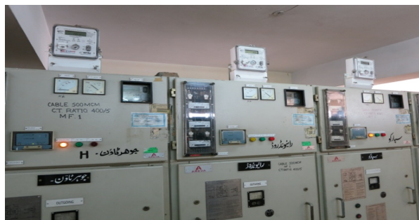
Under the Load Data Improvement Project, smart meters installed at the grid substation feeder panels (left) transmit real-time data about power distributed by Lahore Electric Supply Co. The data appear on screens in the company's newly established control center (right). (Photos by OIG, June 2013)
