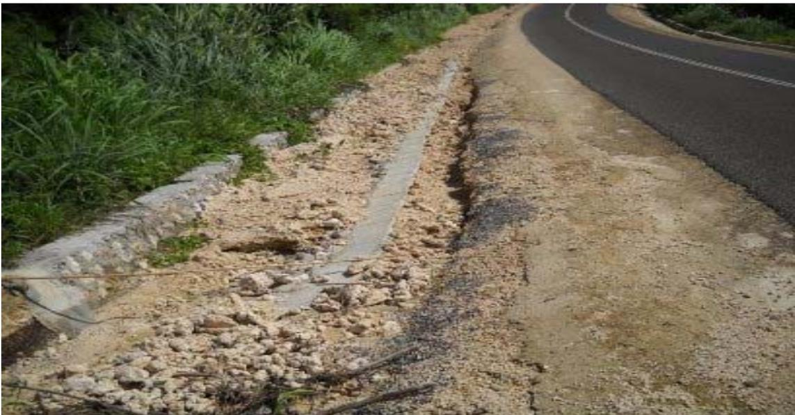
The above photo shows that at the time of the auditors' site visit, a drain on the Efate Ring Road became covered with debris from a failed drain located higher on the hill. That drain failed because of heavy rains. MCC officials subsequently provided us with a photo showing the drain has been repaired. See Appendix II. (Photo by OIG, April 20, 2010)
