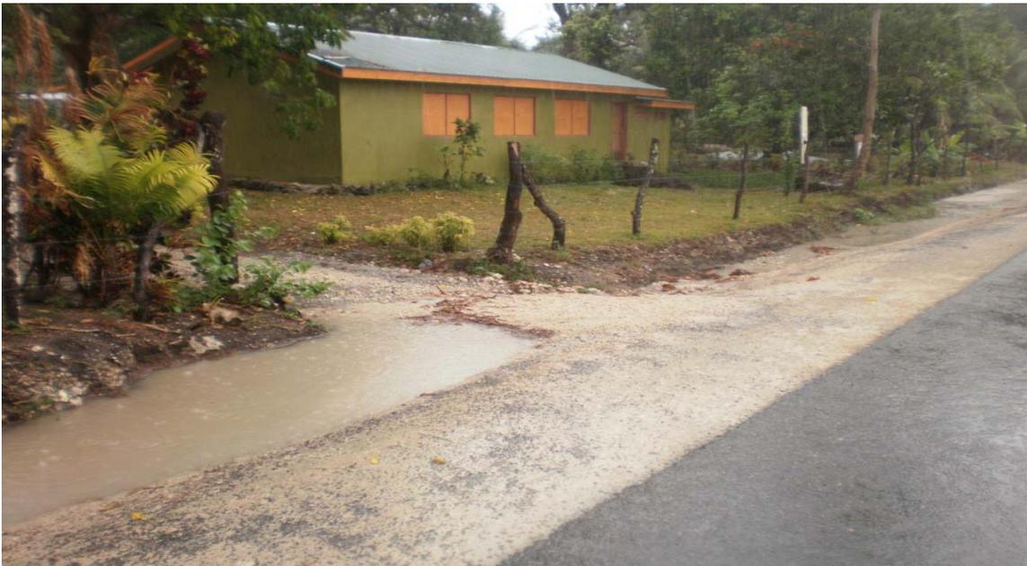
The above photo provided by PWD during the auditors' site visit of the road shows a failed drain pipe on the Efate Ring Road, Tanoliu Village. The drain pipe under the homeowner's driveway was too small and caused flooding of the ditches. MCC subsequently provided us with a photo that the drainage failure has been resolved. (Photo by PWD)
