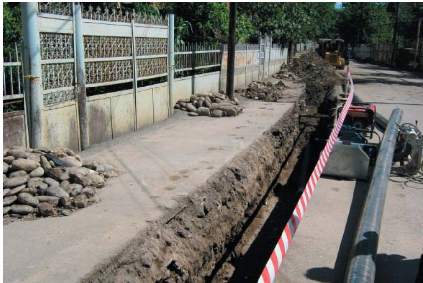
New pipe being laid in Kutaisi, Georgia. (Photo by OIG)
