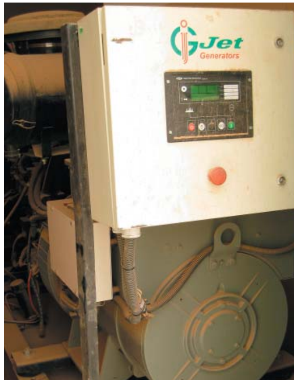
One of two electrical generators, costing $35,000 each, provided under an IRAP grant in connection with an Iraqi rail yard rehabilitation project. (Photo by OIG)
