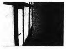
So little thought went into the design and construction of this building that a row of windows was built 6 inches from a wall. As seen here, the windows past the ledge face a wall and cannot be opened.
