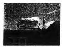
UNDP was told on several occasions that it needed to bolster the structure where water tanks would be located as they can weigh up to 3 tons. The tanks were nevertheless placed on the roof off-line from beams or columns. Structure sections were thus vulnerable to collapse.
