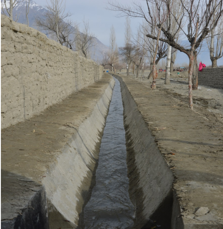
This canal constructed by the project is designed to transport water more efficiently to surrounding areas. Photo: OIG (December 21, 2015)
