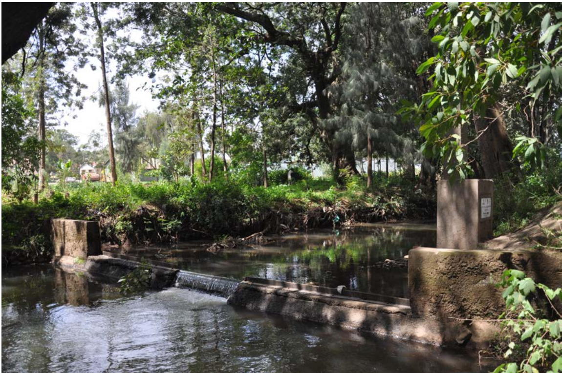
Water flows through the Nanyuki River gauging station in Nanyuki, Kenya. Photo: OIG (June 12, 2017)
