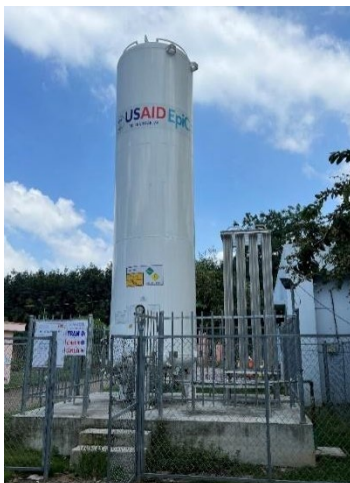
USAID-funded liquid oxygen system located at Long Khanh Regional General Hospital in Dong Nai, Vietnam (photo by Williams Adley).
