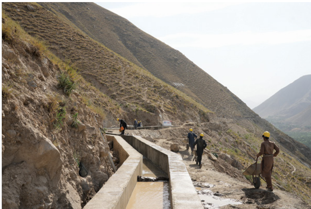
The Korkho irrigation canal under construction in Badakhshan Province. (WFP photo)
