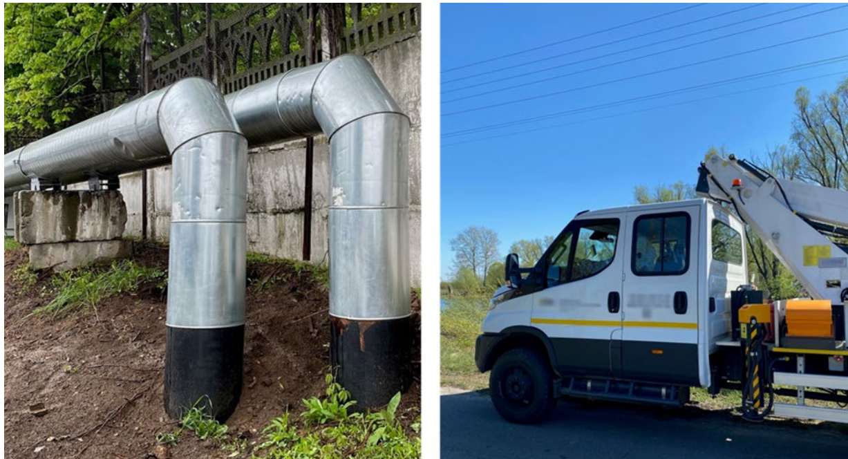
Left: Pipes purchased by Tetra Tech transport hot water in a Ukrainian city. Right: A bucket truck purchased by Tetra Tech supports maintenance work on powerlines next to a rural road in Ukraine. Photo credits: OIG (April 2024).
