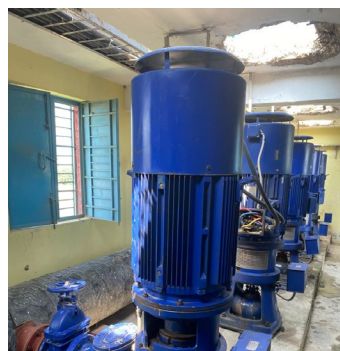
A hole in the water pump room roof leaves equipment exposed to the elements (left), and a nonfunctional latrine shows the unsanitary conditions in a selected school (right).
